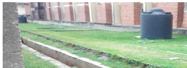
Plate 4.6: Water Facilities close to the Site
