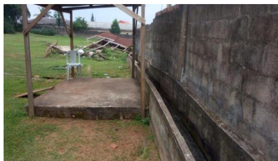
Plate 4.4: Drainage Channel beside the Site
